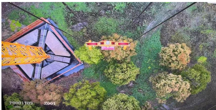
图6 激光雷达与视觉AI实时跟踪吊物轨迹
